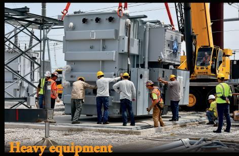
**Above** Corn Belt Power electrical maintenance crews assist crane operators to place the new 84 megavolt-ampere transformer at Burt Switching Station. This transformer has the capacity to power about 54,600 average sized homes. It weighs 120,400 pounds empty and 213,305 pounds once filled with oil.
